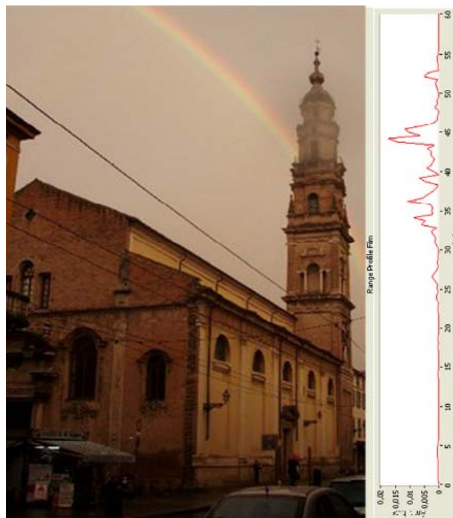
Figure 4. The San Sepolcro tower-bell and the peaks of displacement signal along its height.
